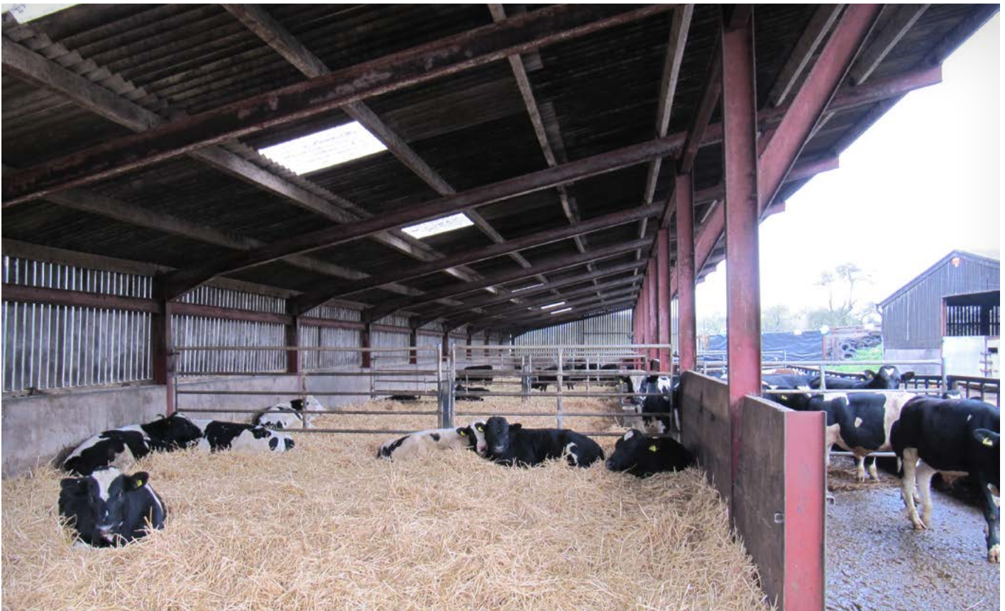
An example of good ventilation
